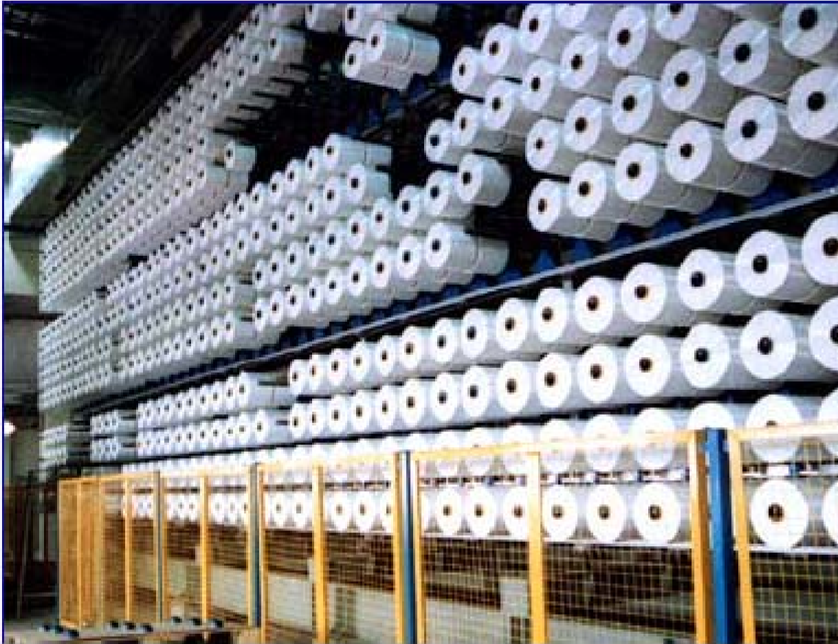
Three-tiered Carousel Tower installed in the existing Hazira Plant
